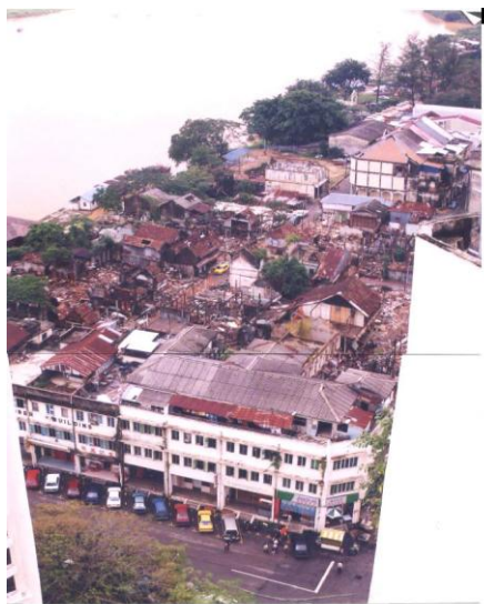
Figure 1: Destruction of old shophouses Source: Wan Ismail & Shamsuddin (2005)
