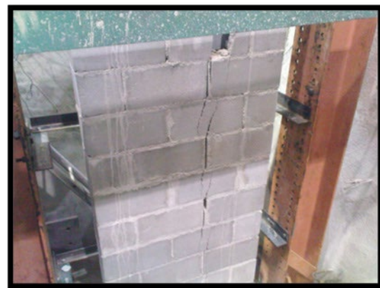
FIGURE 12. Crack due to tensile failure
