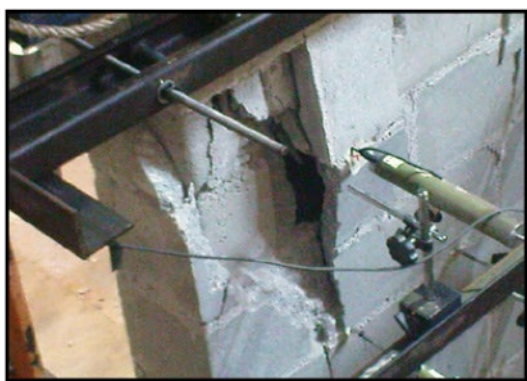
FIGURE 13. Local crushing on masonry
