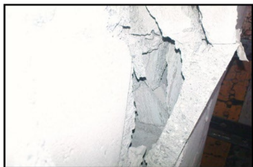
FIGURE 14. The inside of wall view
