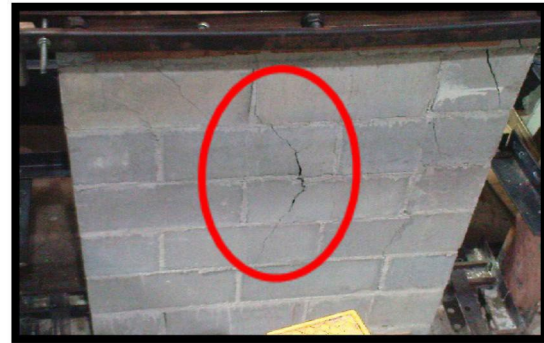
FIGURE 11. Out-of-Plan Crack of Masonry Wall-Column
