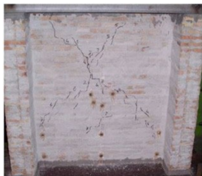
FIGURE 1. Shear cracking damage of HURM wall
