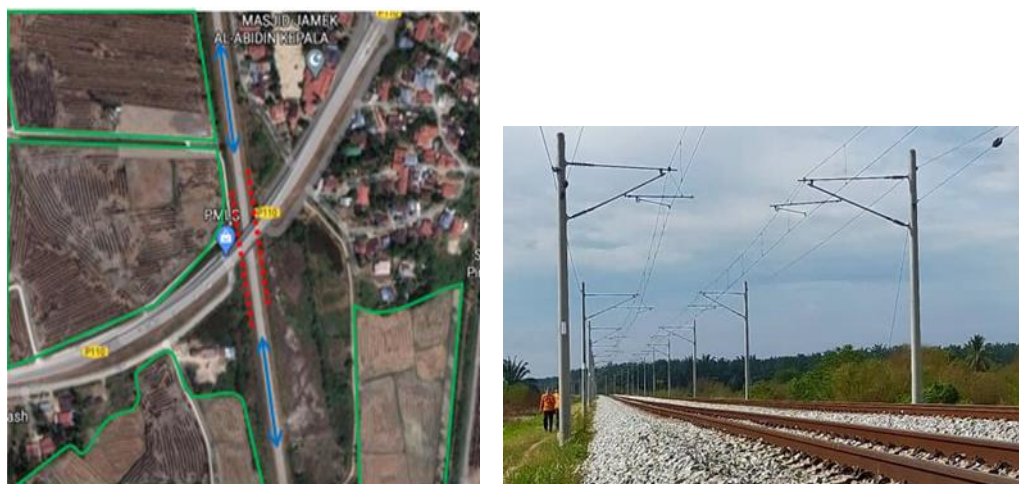
Figure 1: Railway track at Pinang Tunggal (KM 23) Pulau Pinang [17]
