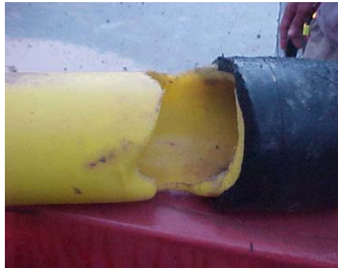
Figure 2 Failed specimen of PE pipe
