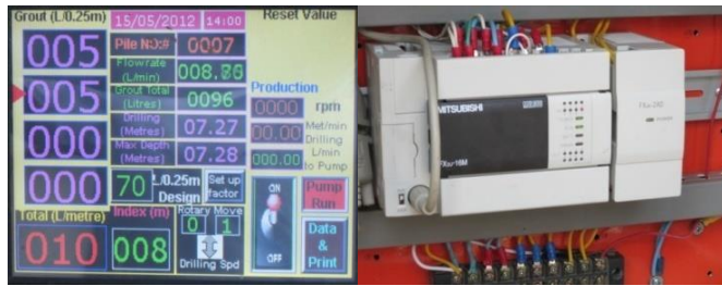
Figure 6 A touch screen displaying operating parameters during the Jet Grouting working
