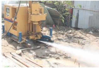
A Grouting machine
