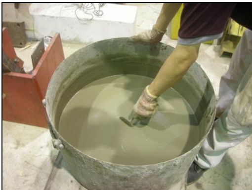
Figure 4 Preparation of grout
