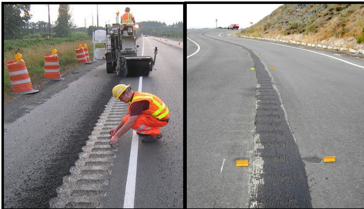
FIGURE 5. the installation of Shoulder Rumble Strip [left] and Centerline rumble strips [right]
